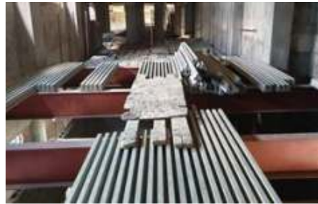
•Steel decking replaced by beam and block
