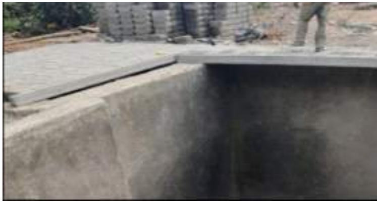
•Underground water tank cover slab
