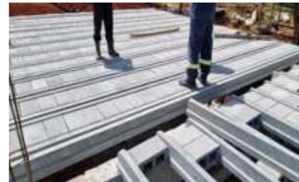
•Residential houses slab installation
