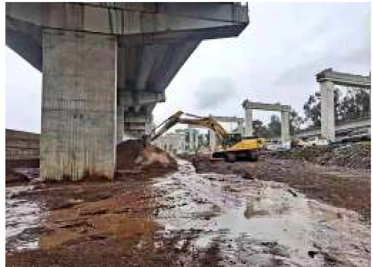
Restoring drainage after heavy rains on Mombasa Road
