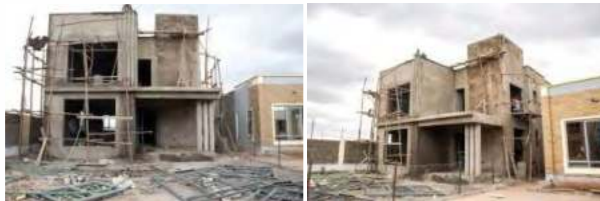
Ongoing construction works on the ground.
