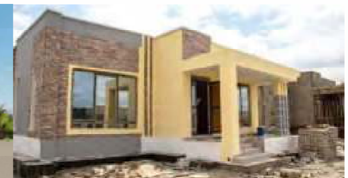
Almost complete unit
