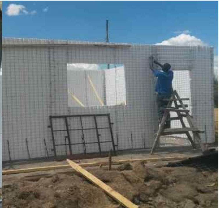
EPS panels, a white foam plastic material made from solid beads of polystyrene, are manufactured in a factory and transported to the site for assembly, which
