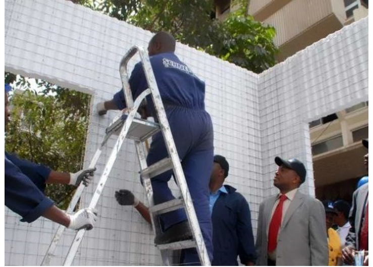
EPS panels, a white foam plastic material made from solid beads of polystyrene, are manufactured in a factory and transported to the site for assembly, which
