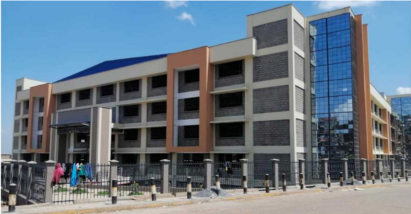
MODERN MARKET, NGONG TOWN, Kajiado County. Client: NAMSIP (Nairobi Metropolitan Services Improvement Program) Project Complete
