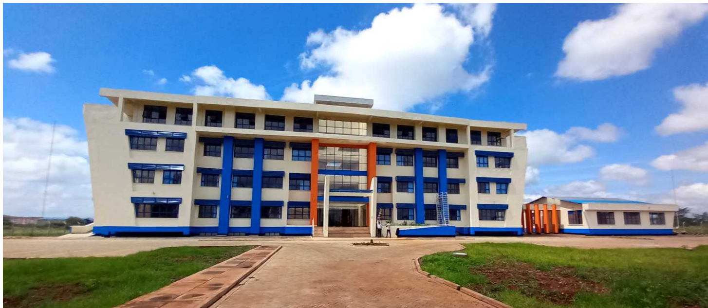
AREA CONTROL & DISASTER RECOVERY CENTER , Mlolongo, Machakos County. Client: KCAA (Kenya Civil Aviation Authority) Project Complete
