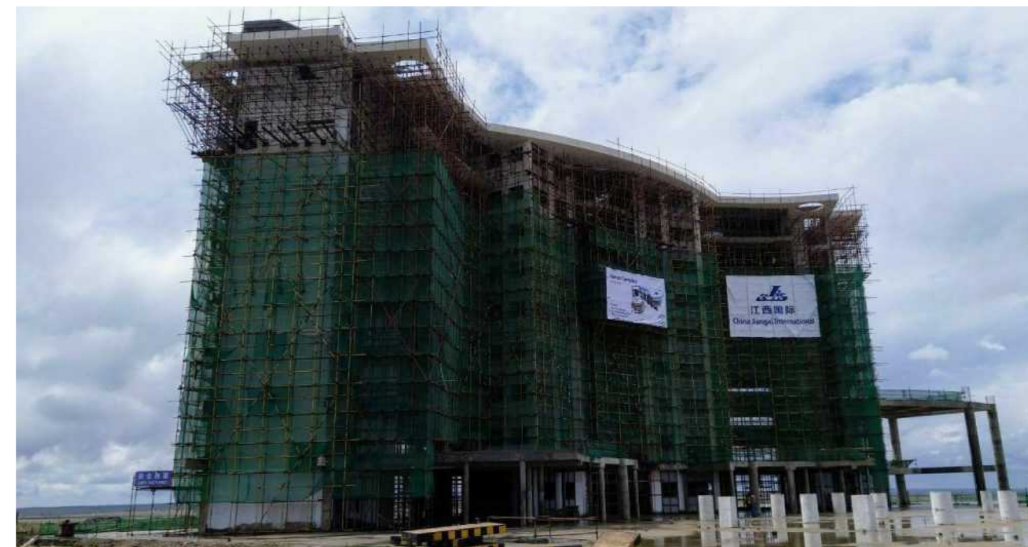
Konza National Data Center - under construction
