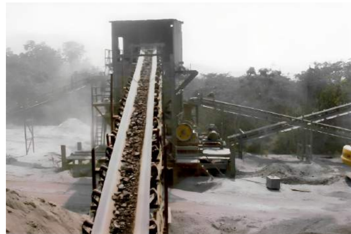
Conveyer Belts & Crush Plant
