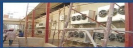
HVAC INSTALLATION AT MTN KANO
