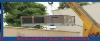
INSTALLATION AT ROCK CHRISTCHURCH, ORAGADA LAGOS
