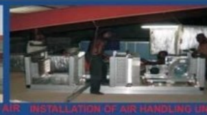
INSTALLATION OF AIR HANDLING UNIT AT THE METROPOLITAN CLUB LAGOS
