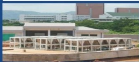
COURT OF APPEAL HQ AND ABUJA DIVISION, ABUJA
