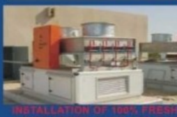
INSTALLATION OF 100% FRESH AIR UNITS AT MTN KANO AND IBADAN
