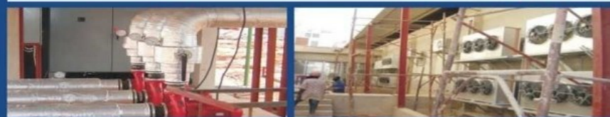
PRIMARY PUMP INSTALLATION AT NIGERIA JUDICIAL COUNCIL
