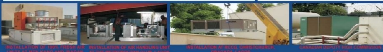
INSTALLATION OF 100% FRESH AIR UNITS AT MTN KANO AND ISADAN
